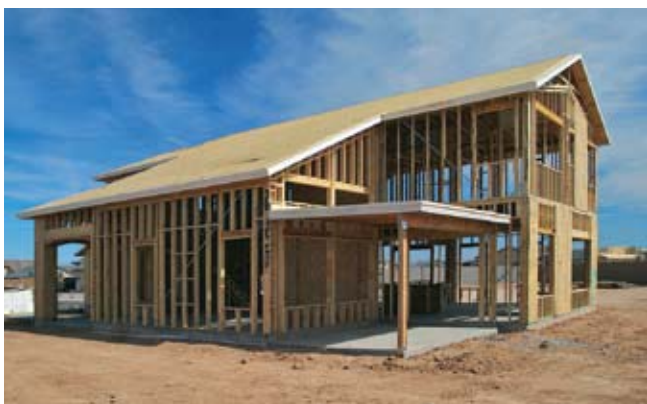
Construction of new homes in Phoenix, Arizona.
